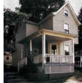
Morgantown Homecoming renovation at 222 Cherry St., in Greenmont.
